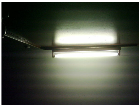
The “beat effect” problem created when shooting photos under standard fluorescent lighting
