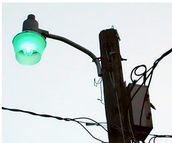
A 175-watt mercury-vapor yard light approximately 15 seconds after starting
