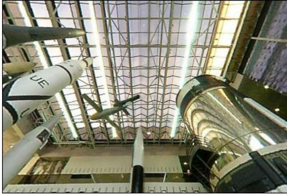
Sulfur lamps with light pipes on the ceiling of the U.S. Air and Space Museum in Washington, D.C.
